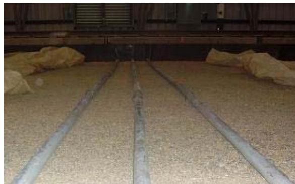
FIGURE 8. CONDUIT SET-UP FOR INSTRUMENTATION WIRES
