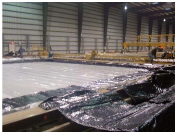
FIGURE 14. PLACEMENT OF POLYETHYLENE SHEETS AND BLANKETS
