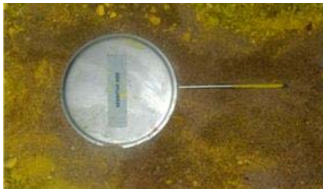
FIGURE 5. INSTALLED SOIL PRESSURE GAGE
