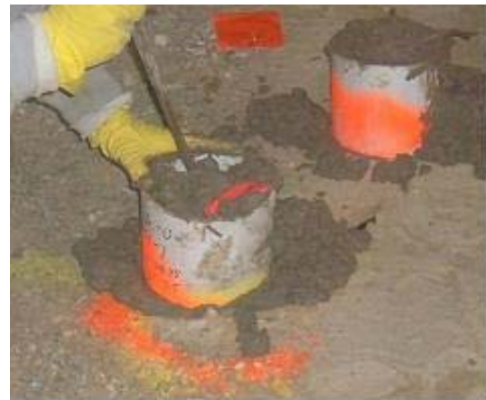
Placing concrete into cans
