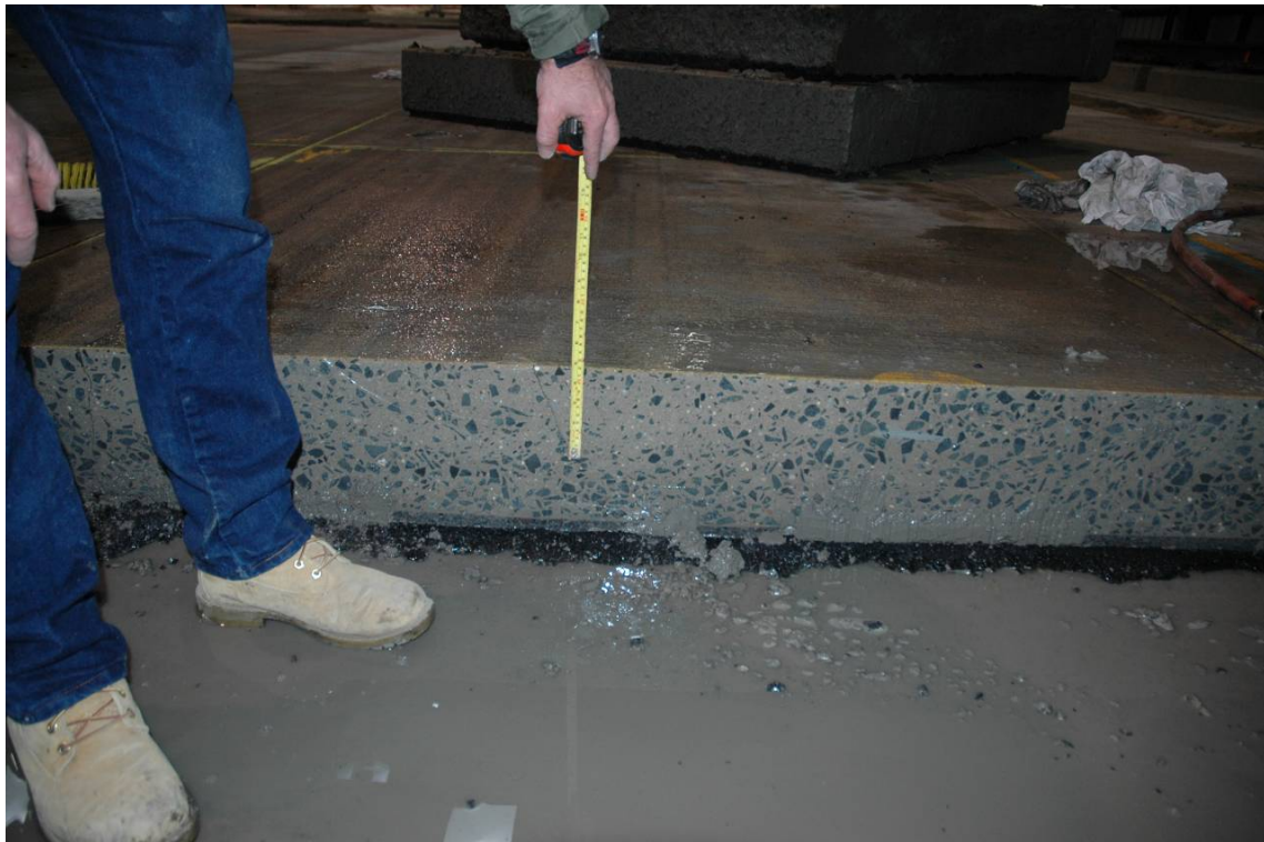
FIGURE 42. TOP-DOWN CRACK VISIBLE AS OVERLAY SLAB BENDS DURING REMOVAL
