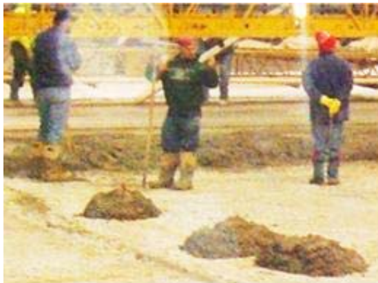
Instrument cans piled with concrete
