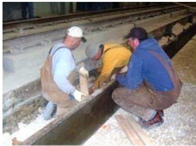
FIGURE 7. PLACING SIDE FORMS
