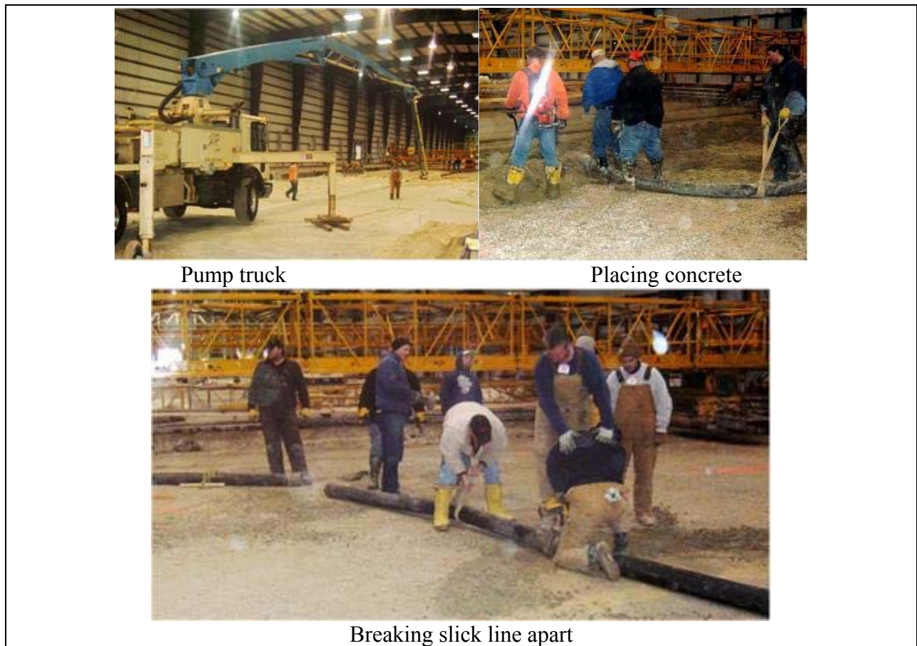
FIGURE 12. PLACING CONCRETE FROM SLICK LINE
