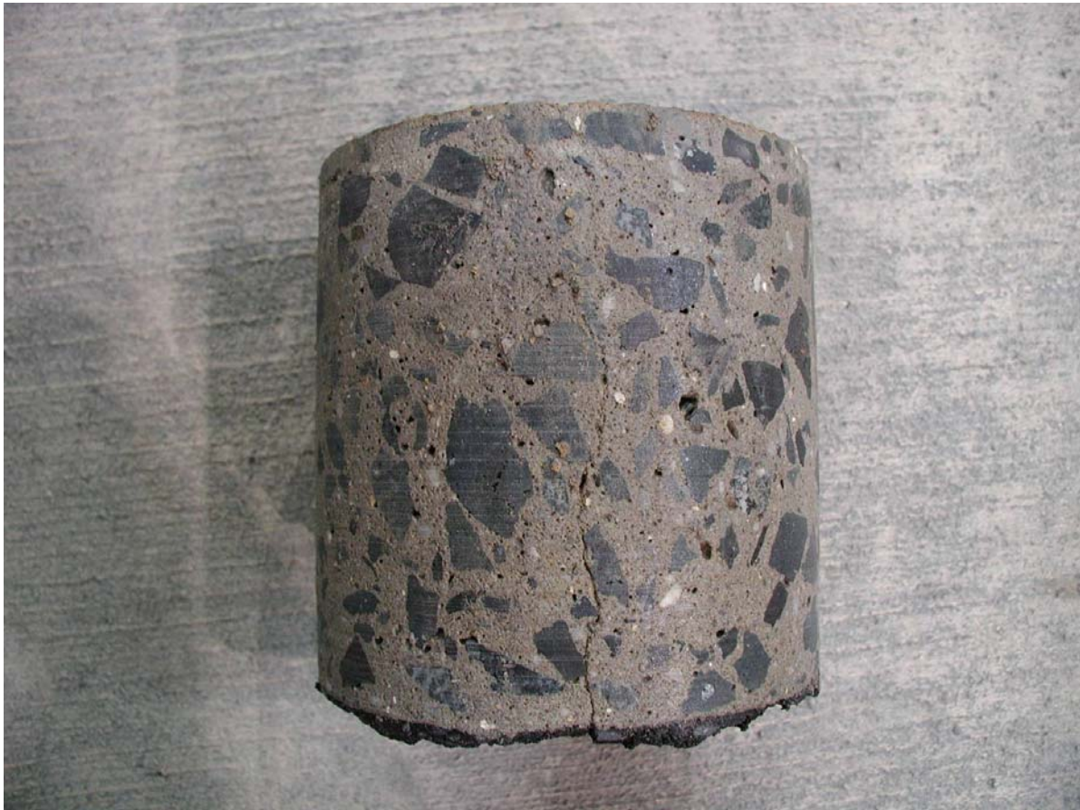
FIGURE 40. CORE FROM TRANSITION 5 SHOWING BOTTOM-UP CRACK THAT HAS NOT PROPAGATED TO THE SURFACE
