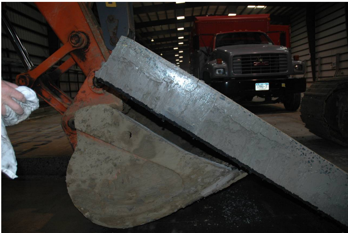
FIGURE 41. OVERLAY SLAB REMOVAL WITH ASPHALT INTERLAYER ADHERED AND VISIBLE TOP-DOWN CRACK
