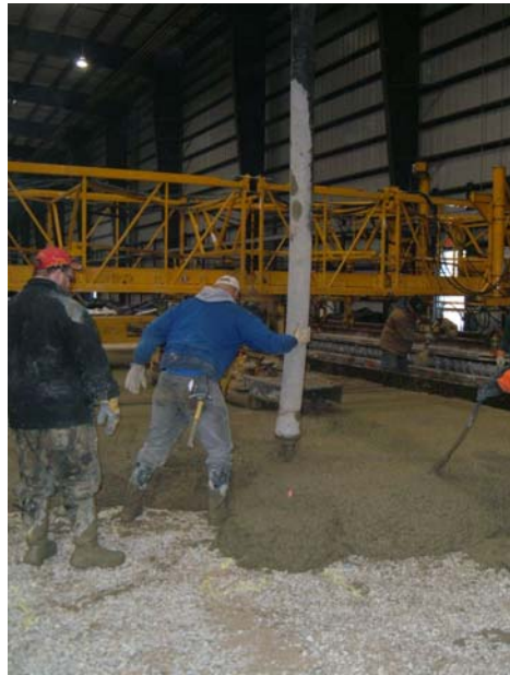
FIGURE 13. PLACING CONCRETE WITHOUT A SLICK LINE
