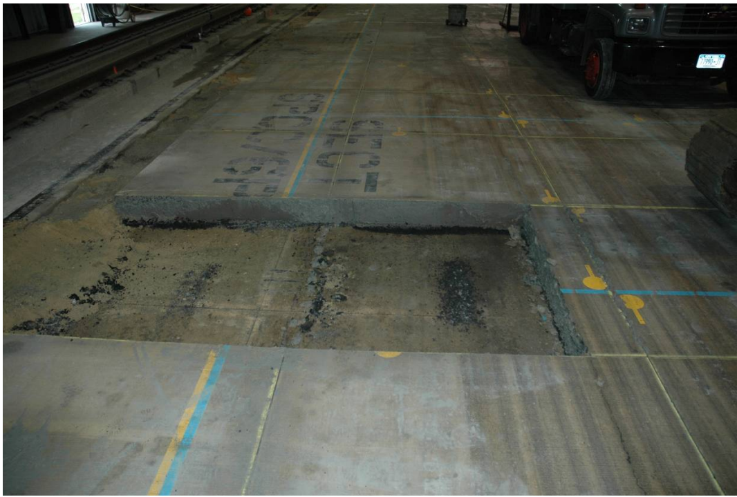
FIGURE 44. CRACKS OFFSET FROM LONGITUDINAL JOINT IN TEST ITEM N1
